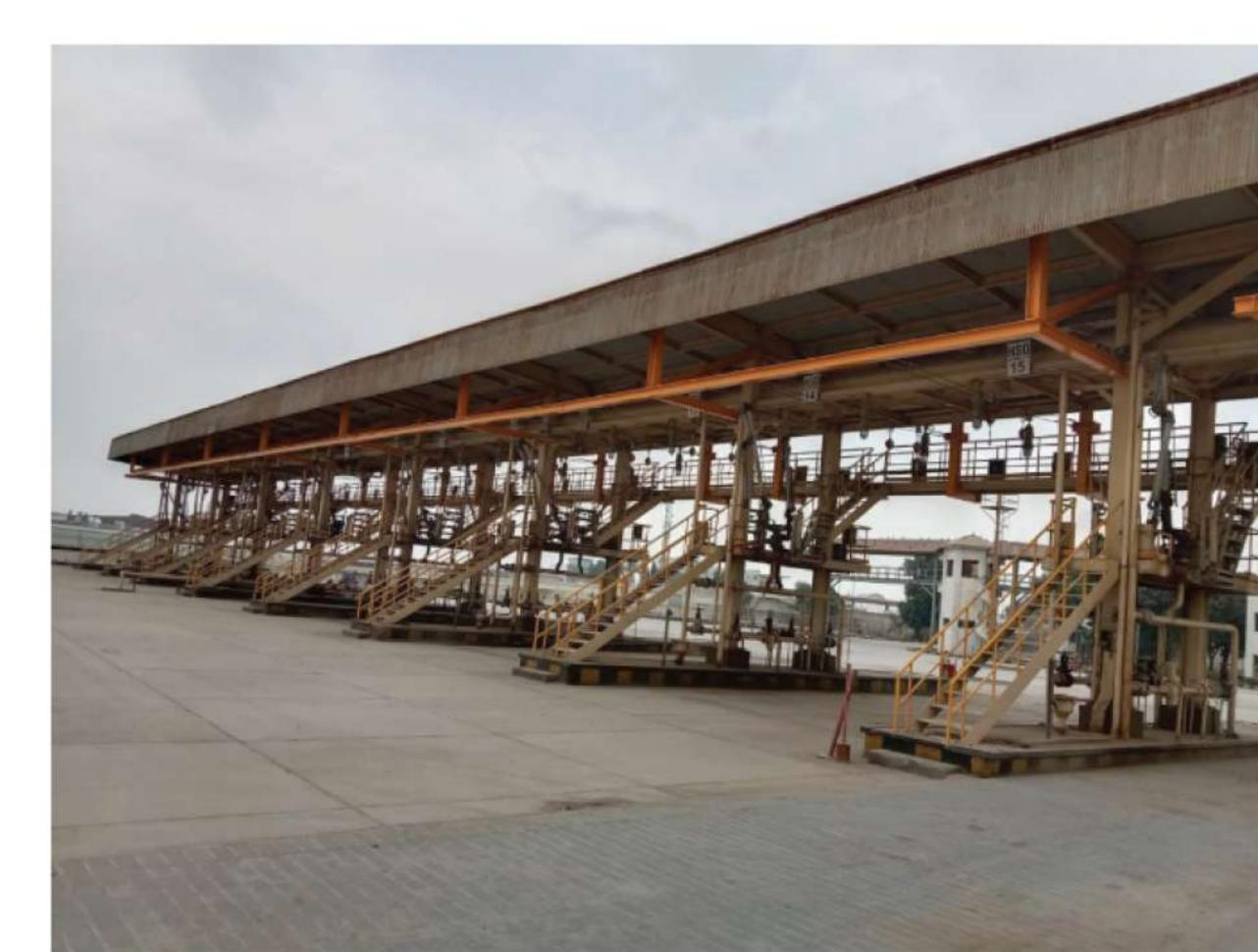
Owing to Operational limitations of welding the new structure at the gantry, the fall arrestor system at these locations has been designed based on the bolting of the structure.
