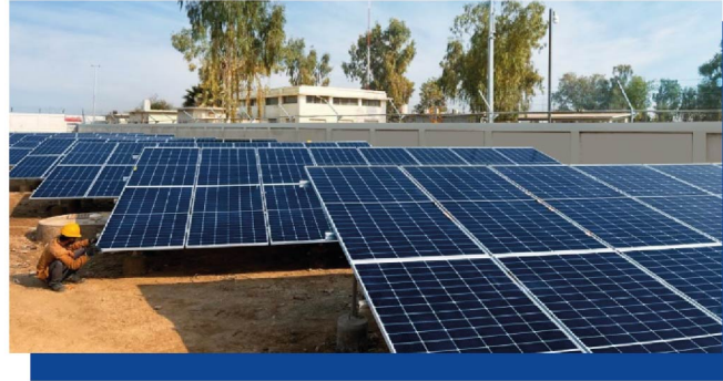
1 st renewable Solar Power Plant commissioned at Shikarpur Terminal with a potential capacity of 200 KW and a production of 345 MWh per annum.
