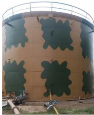
Rehabilitation of Tank at Sihala
