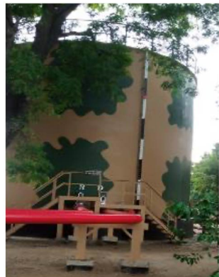
Construction of Fire Water Tank at Habibabad
