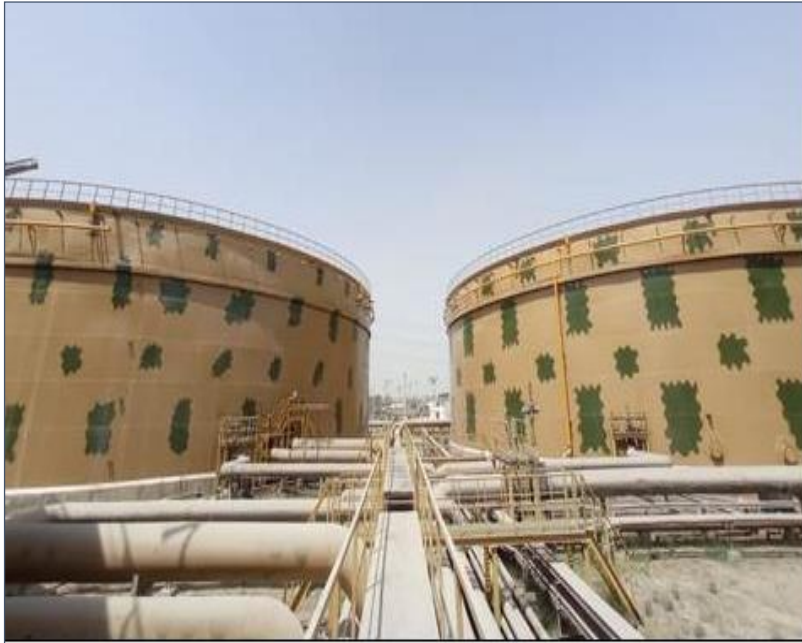
79 thousand tons of existing storage has been rehabilitated in FY23
